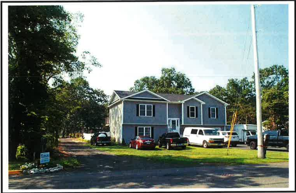
Subject (impacted) Property – 61 Bailey Road, North Haven
